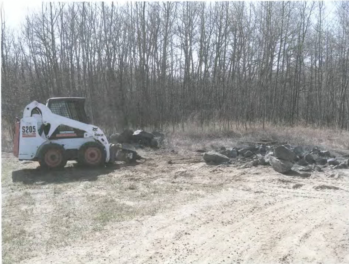
SKID STEER LOADER WITH HYDRAULIC HAMMER AND BREAKER POINT - LARGER BOULDERS IN BACKGROUND
