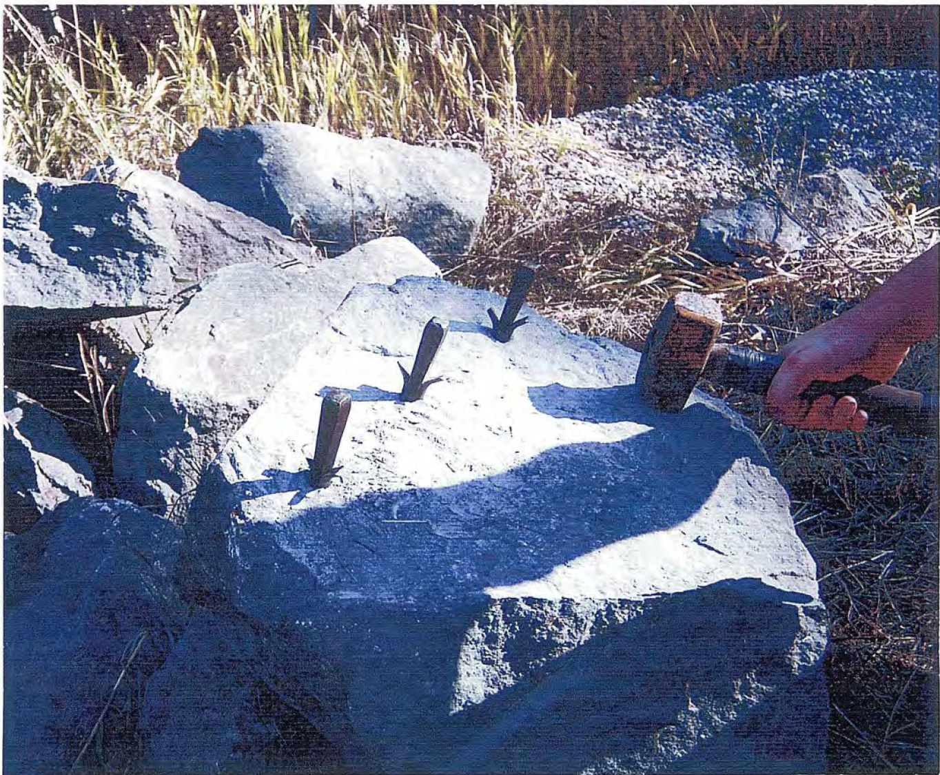
Fig. 6 – “Feathers and Irons” being used to split large rock
