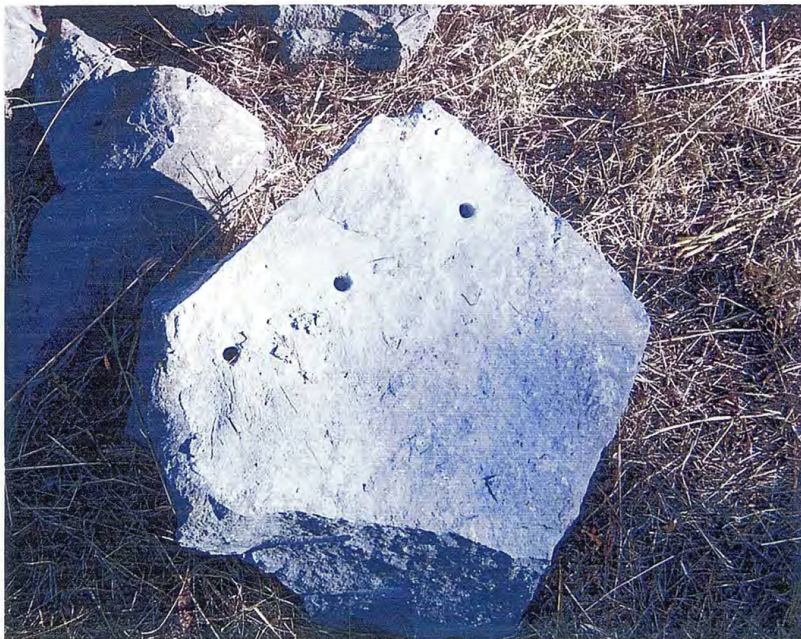
Fig. 20 – Holes are drilled in large boulder
