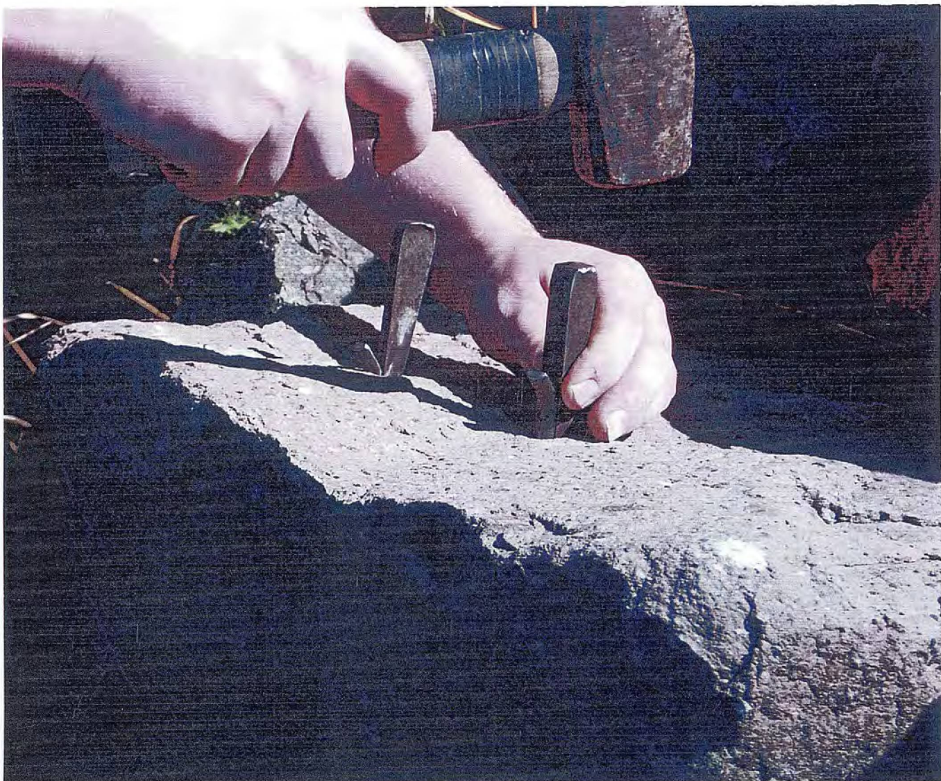
Fig. 22 – Placing Feathers and Irons
