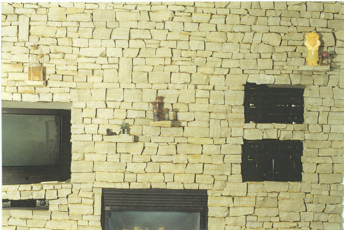
Photo 7. An interior wall clad with the Bighorn Sandstone. Note: The colour of the stone on this photograph is too yellow.
