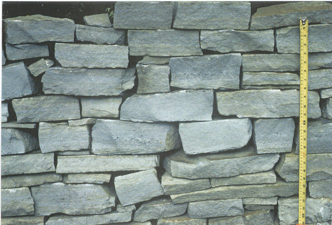
Photo 6. Typical dimensions of the Bighorn Sandstone used as a dry-pack wall stone. Note: The colour of the stone on this photograph is too blue.
