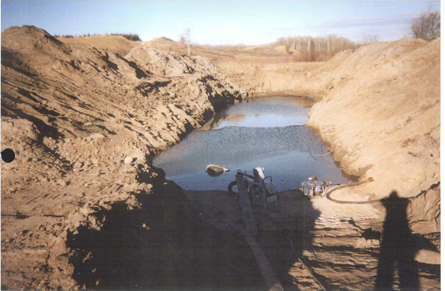
GROUND WATER SETTLING POND BEHIND SIC PLANT
