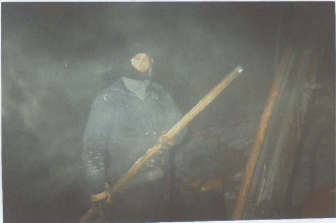
Drilling in progress
