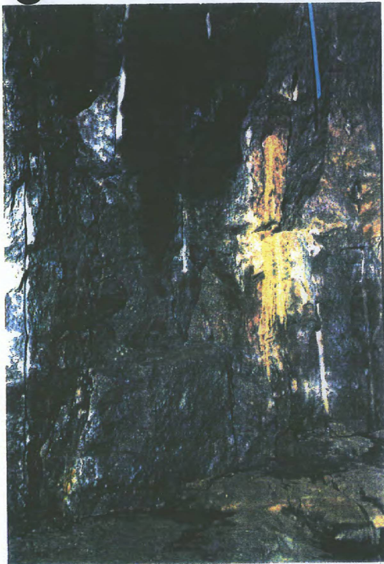
Photograph 9. Active quarry face, shows detail on R.H.S. of photograph 7; note good separation along the intensely oxidized (rusty) subhorizontal fracture at base of the quarry face; discontinuous, subhorizontal parallel fractures form small ledges; a zone of closely spaced vertical shear fractures are at the extreme L.H.S. of the photograph; drill holes and wet areas (dark) mark the quarry face.
