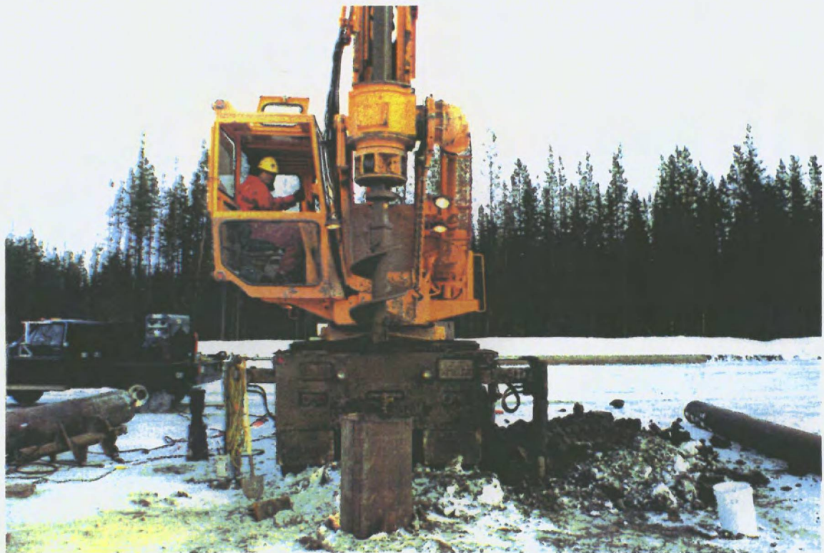
Photo 2. Rat Hole Drill Rig at Drill Site "C"
