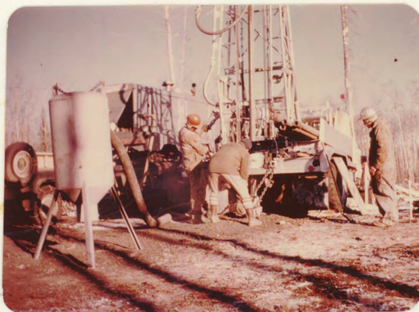
Air Separator and Compressor at left. Operator collecting cuttings with screen.
