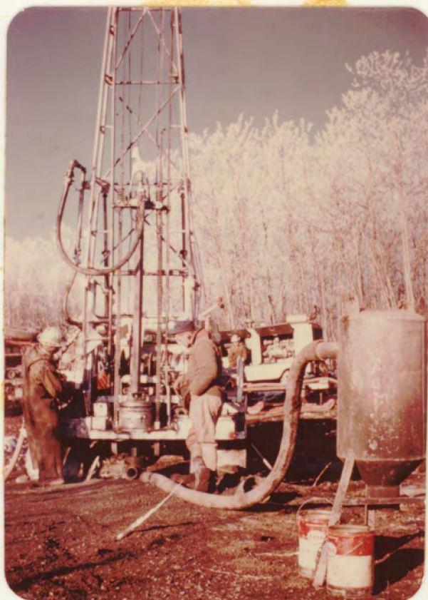
View showing orifice at top of "sealing head". Samples collected in buckets shown beside separator.
